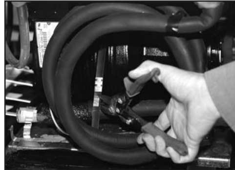
Cutting band that is around compressor
